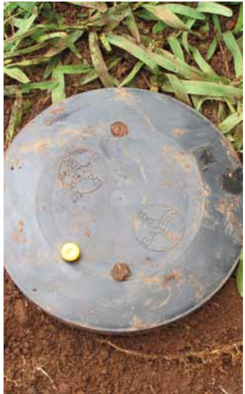
Holes 'mudded up' confirming termites are present in the In-Ground Station.
